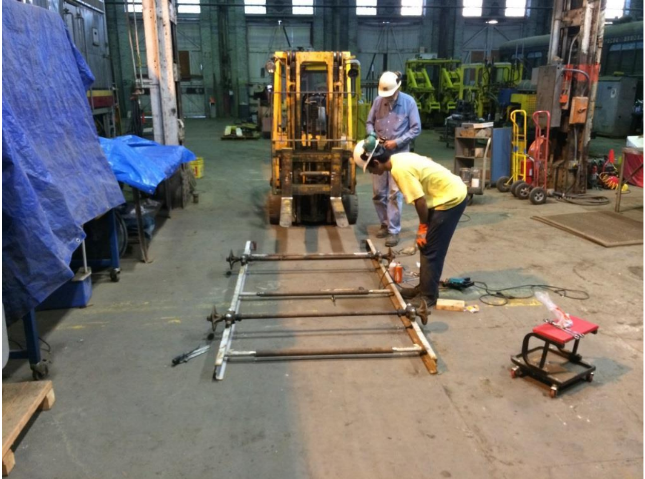
Alan and Josh work on building the frame for the new MOW flatcar
