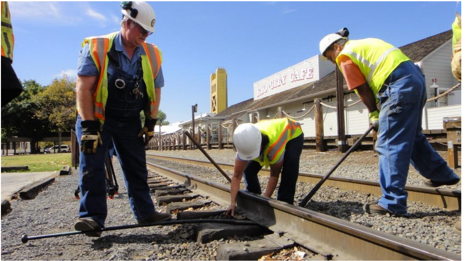
While there, we dealt with some minor maintenance issues. We replaced a tie-plate that had become dislodged. Chris and John nip the rail as Pam puts the tie-plate back into position.
