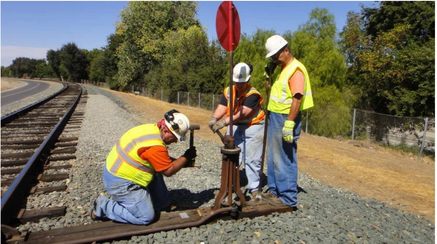
Mike F., Heather, and John stabilize the wobbly switch stand at Switch 17
